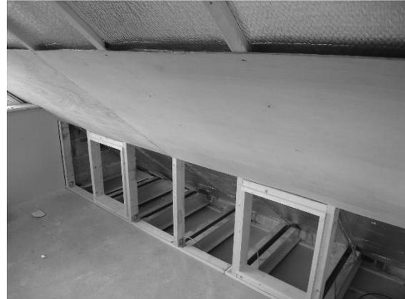
Check integrity of existing lateral restraint straps to ensure they are still functioning correctly and secure to trusses/ashlar stud, walling and flooring.
